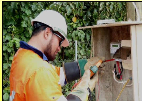
Installation of new meter before connection of power supply.
